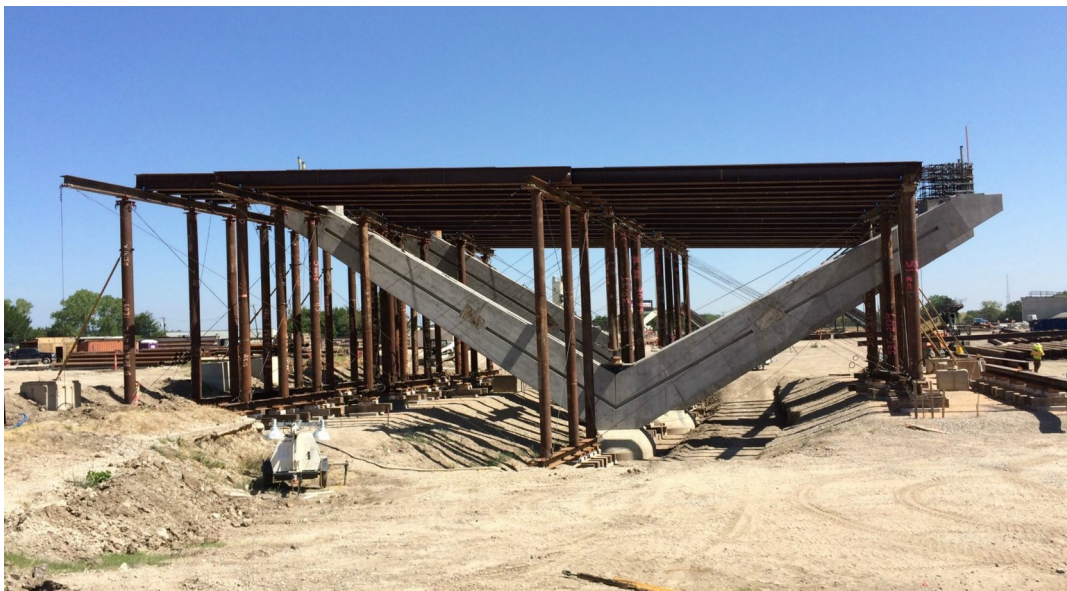
(White Settlement V-Piers for bridges under construction)
