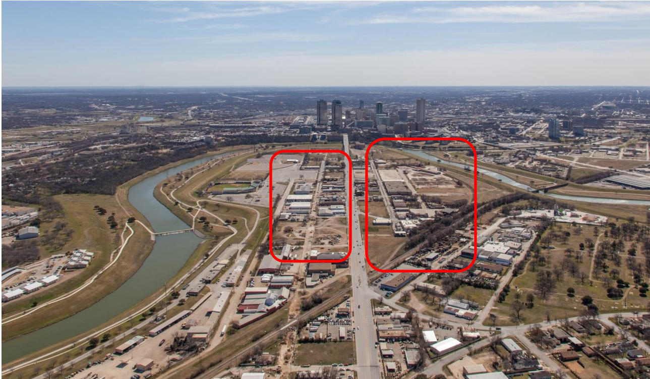
(North Main Street aerial after relocation, demolition, and environmental work)
